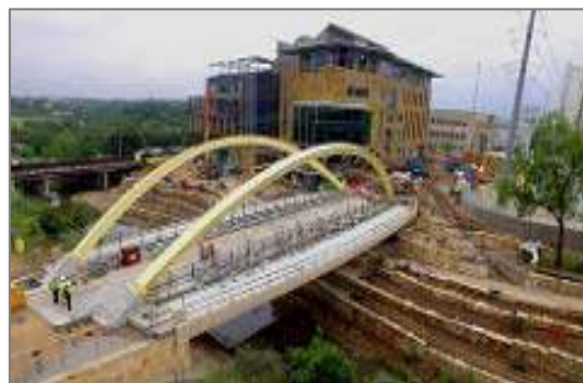
New Central Library Construction 2016
