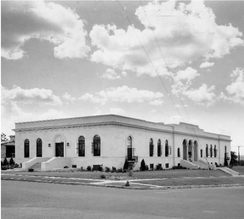
Figure 1. Original AHC Exterior View_Photo by COA
